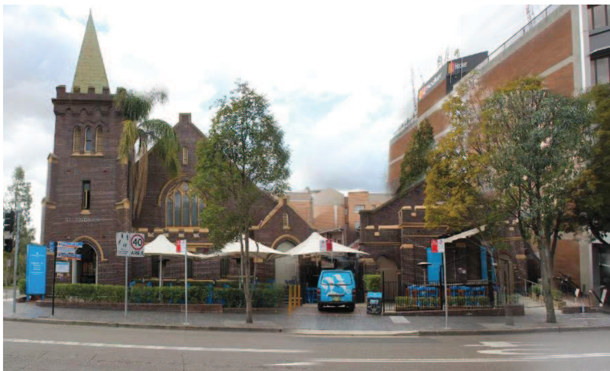
Fig. 1 St Andrews Uniting Church and Margaret Houison Memorial Hall in Phillip Street
