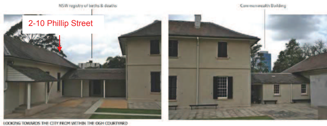
Figure 15: View 1B - approximate location of the subject development site is indicated
