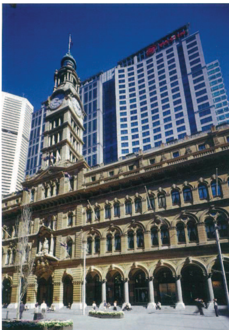
Fig. 3 GPO Western Hotel, Martin Place
